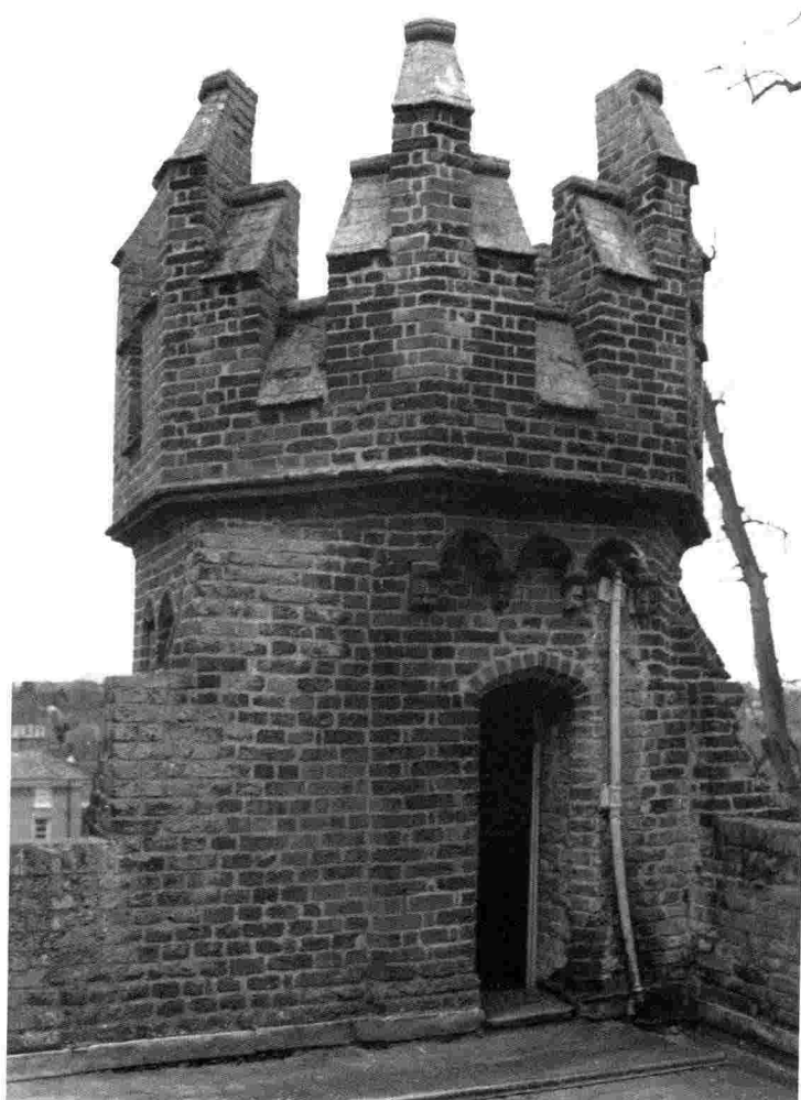
FIG. 2 – The dovecote from the east ( photo: author ).
