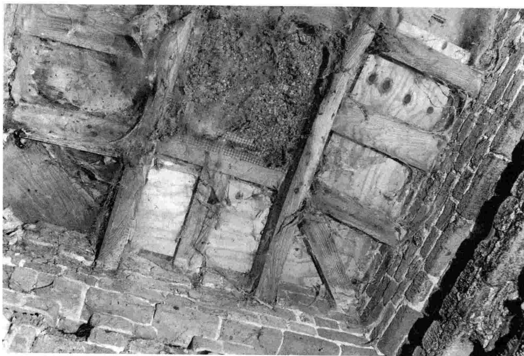
Fig. 5 – The roof structure from below, showing the rectangular aperture through which the pigeons formerly entered ( photo: author ).
