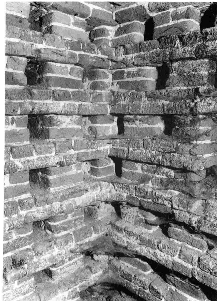
FIG. 3 – The north-west corner, showing the nest-holes and alighting ledges ( photo: author ).
